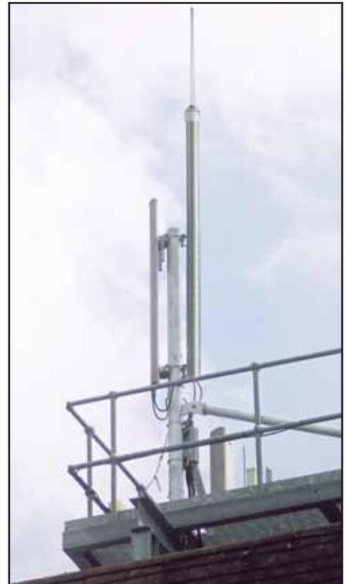
Illustrators representation of installed ERITECH Isolated Downconductor system
