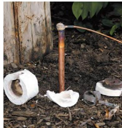
1. After preparing the ground rod and wire, position the Cadweld One Shot and attach the lead to the control unit.
